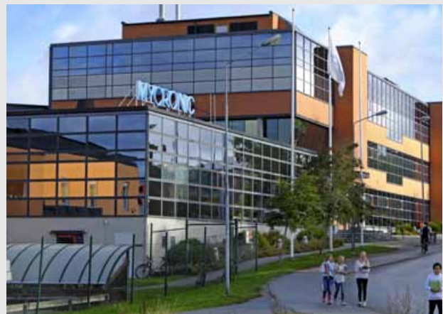
Mycronic's facilities in Täby outside Stockholm. Here several projects have been conducted to decrease the environmental impact of its operations, for example the installation of geothermal heating and a continuous change of light sources to LED.
